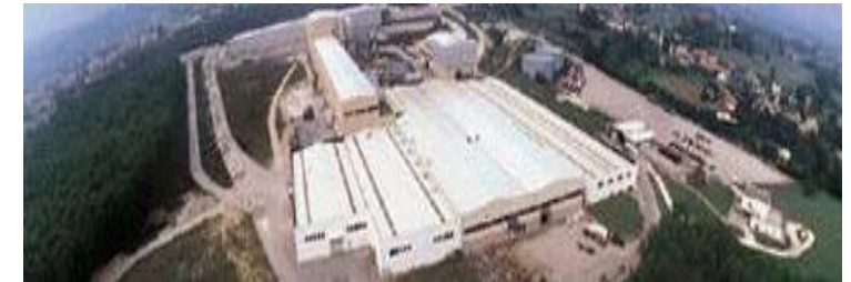
Santa Giustina plant
